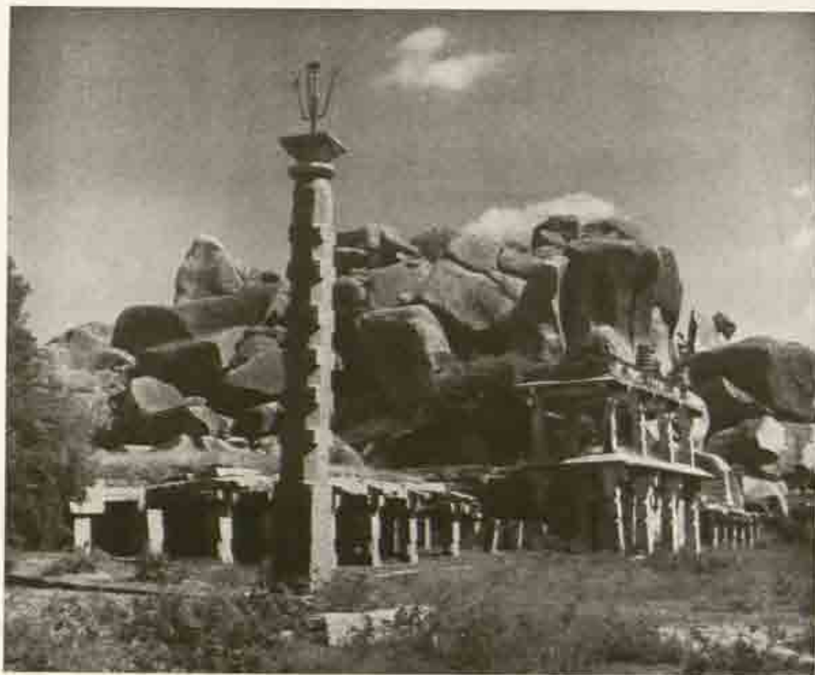
Plate 124. A general view of Temple at Hampi, Vijayanagar: 1513-1542 A.D.
