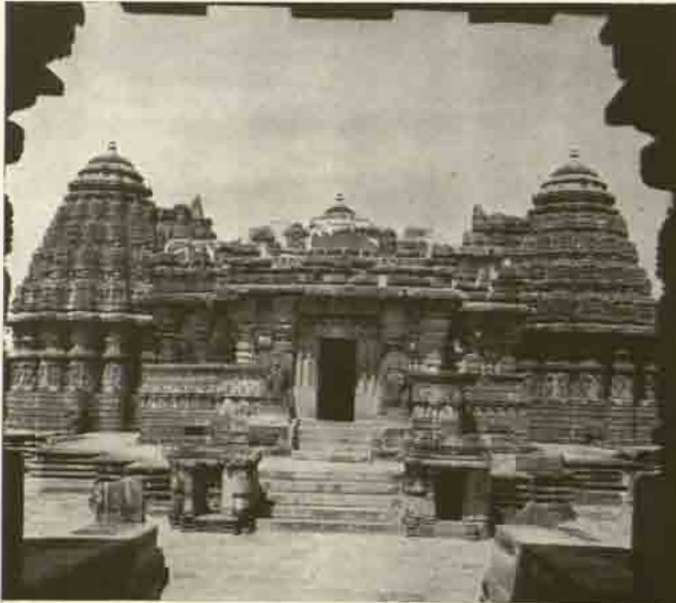
Plate 105. A general view of Somnathpur Temple, Mysore: Showing Hoysala architecture: 1268 A.D.
