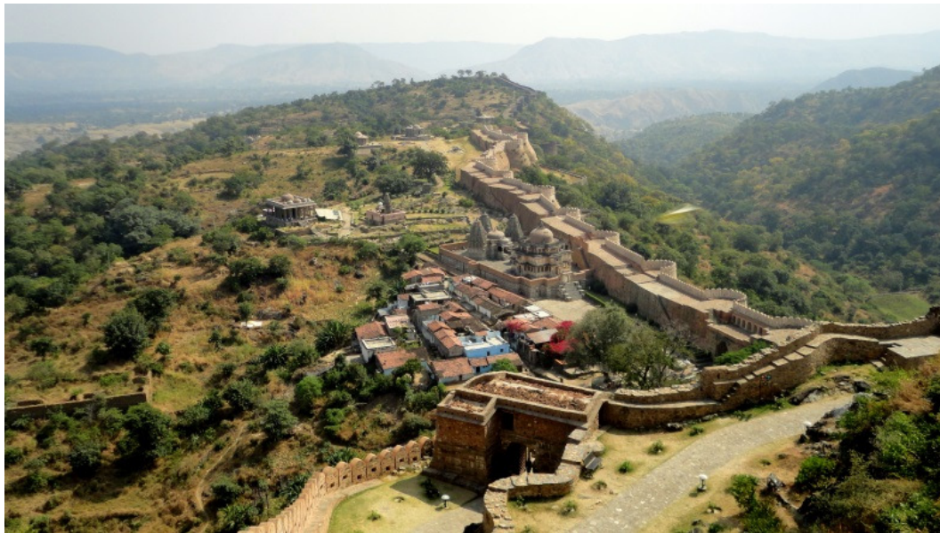
Top: The walls of the fort of Kumbhalgarh extend over 38 km. Bottom: Aerial view of Kumbhalgarh fort (source: Wikimedia commons)
